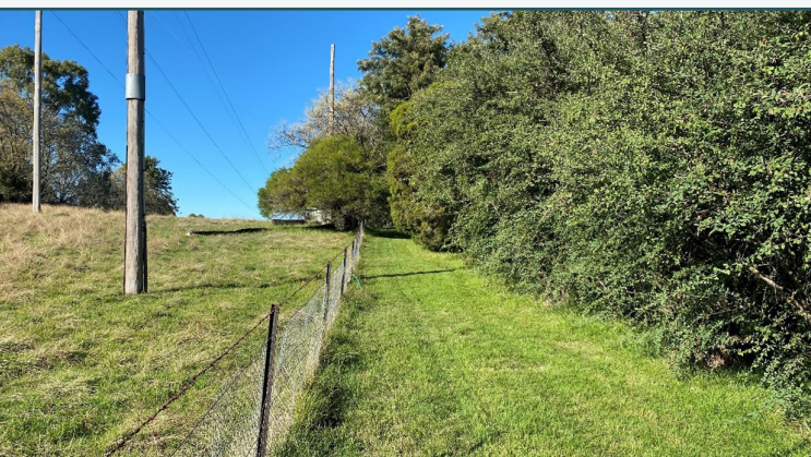
Existing Transgrid transmission line in the proposed site
